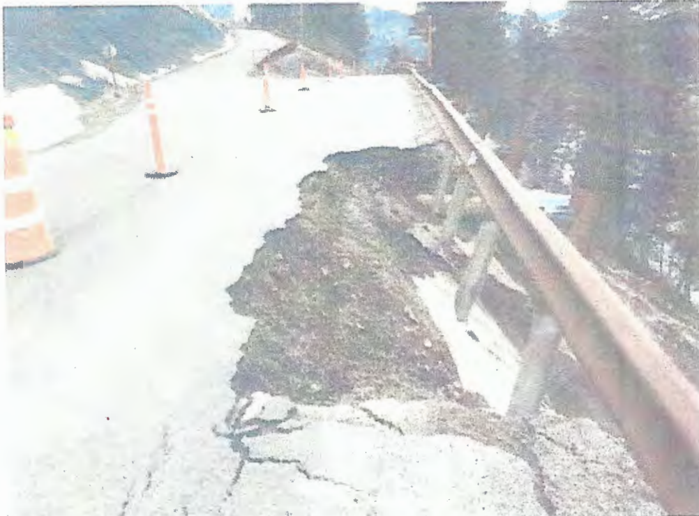
Existing Roadway Condition @ STA 2+50 Looking Southeast – April 10, 2017
